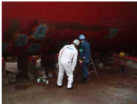
Photo 11. NK is surveying welding
